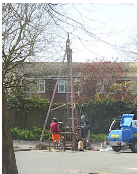
Pile driving in the car park, 19 April
