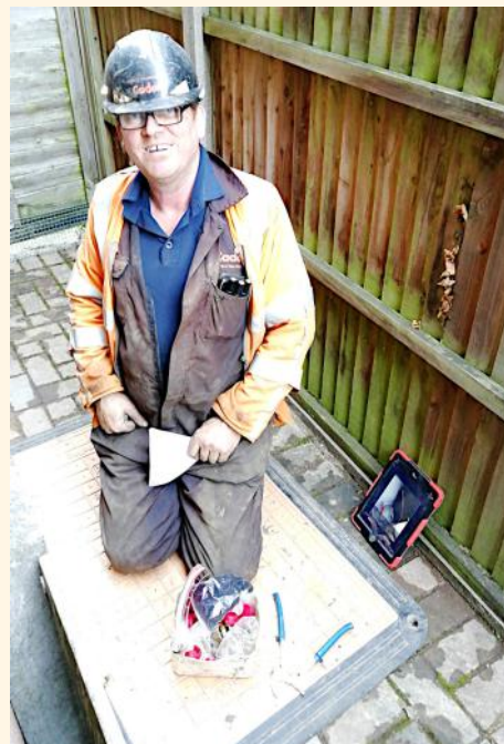
Mike restores the gas supply
